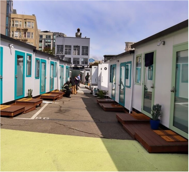
San Francisco & Santa Barbara build faster on parking lots.
